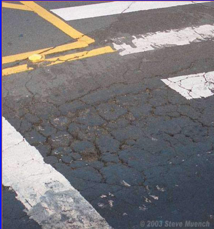
Alligator Cracking
