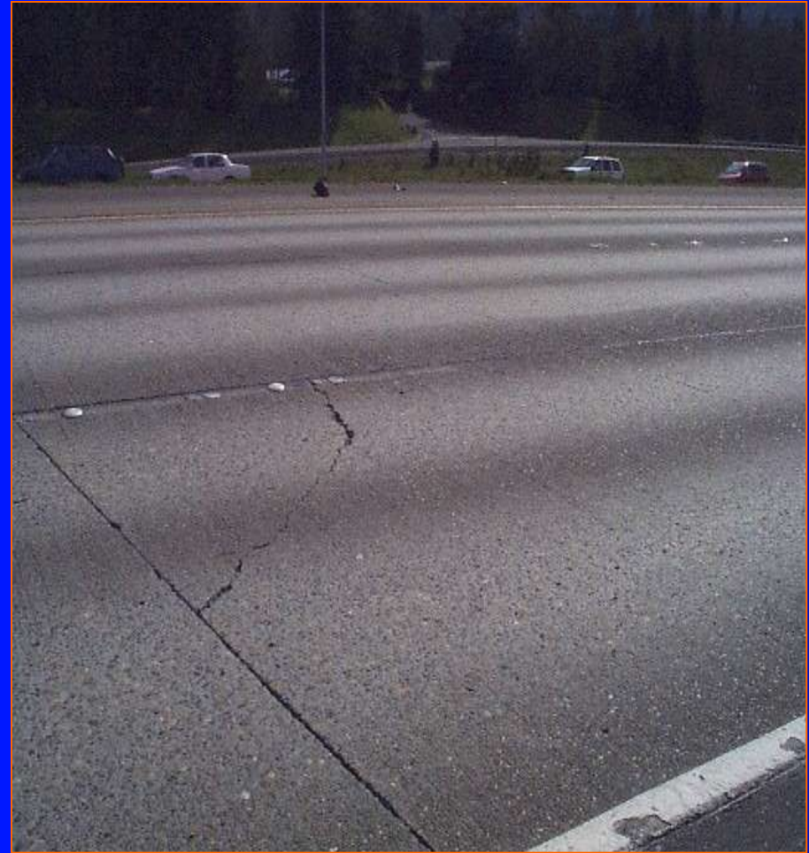
Corner break on a highway
