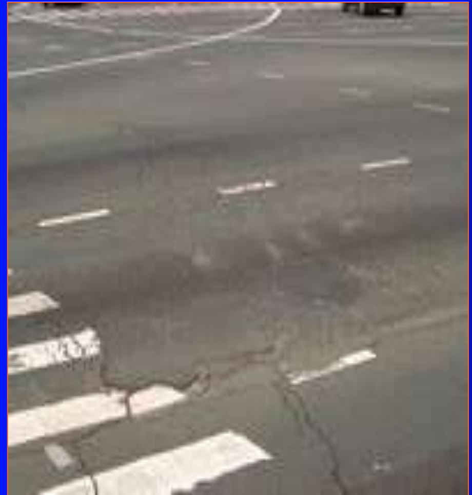
Alligator Cracking
