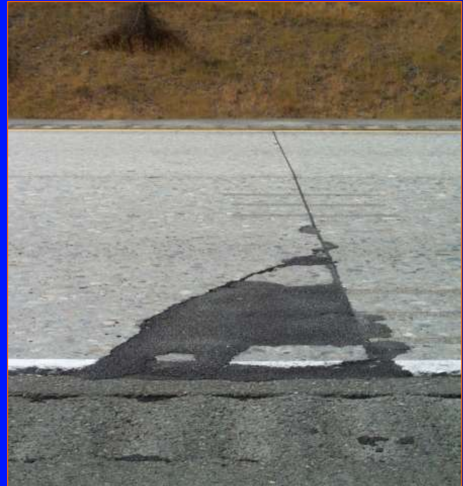
Patched failure
