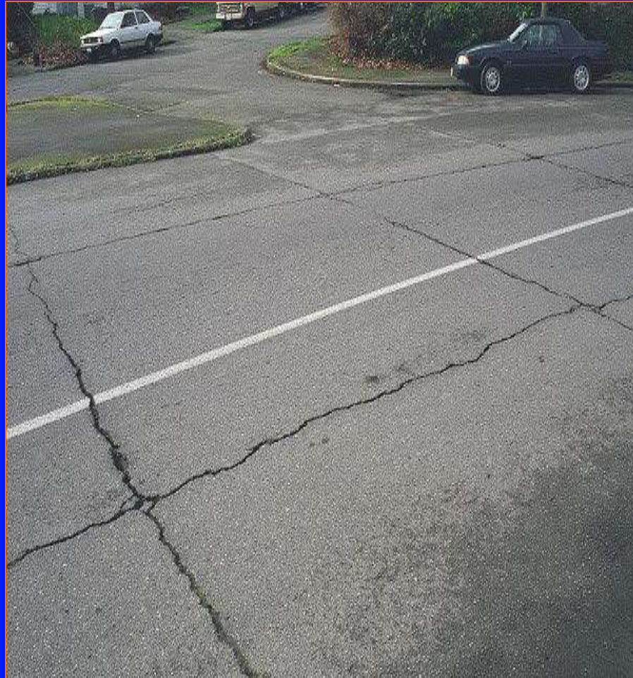
Joint reflection cracking
